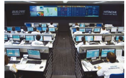
Building equipment is monitored remotely from a call center
