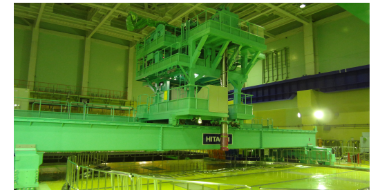
Seismic reinforcement work on fuel handling machine
