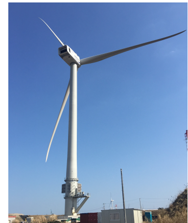
Fukushima wind power station in Kashima, Japan (5MW)
