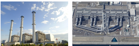
Preventive maintenance for GTCC *4 power plants
