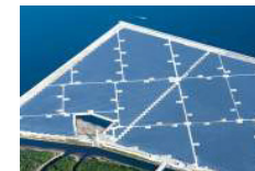
Photovoltaic power generation systems*5
