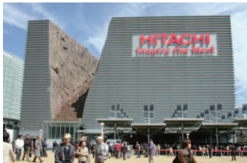
The Hitachi Group Pavilion Exterior
