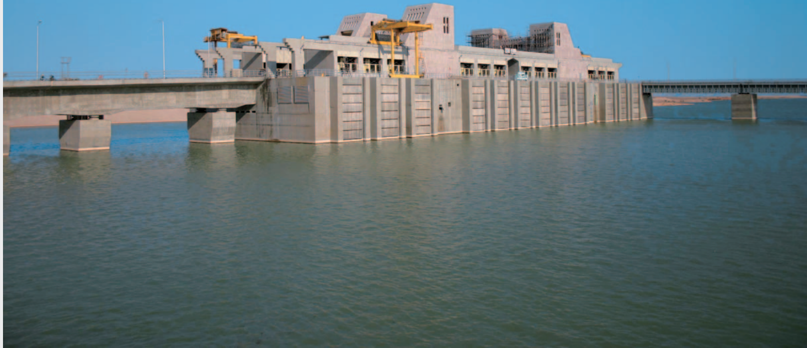
Mubarak Pumping Station
