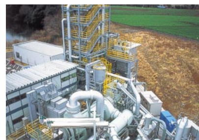
Pilot waste treatment plant using the kiln-type waste thermolysis system in Hitachinaka City, capable of processing 20 tons of waste material a day
